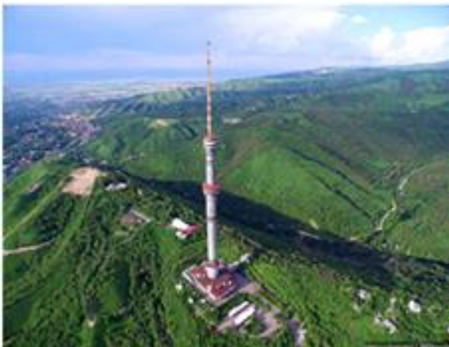
Fig. 1. TV tower erected on top of the landslide dangerous Kok Tobe Mountain in Almaty, Kazakhstan [7]
